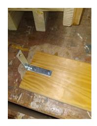
a) Screw the L bracket to the top of part 10 at one end. This will be attached to the post later.
