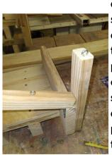
c) Using two eye screws, with the eye opened up just enough to allow the spring to pass through the opening, attach the spring by putting one eve into the top end of part 5 and the other into the top edge of the swing arm (part 6) about one third to one half of the way up the swing arm adjusted accordingly to the spring you are using.
