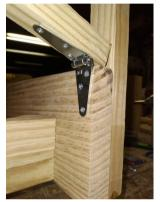
b) Attach the small hinge to part 6, the swing arm, %" from the end of part 6. Then screw the other side of the hinge to the left side of part 4 (the right side piece of the jug base) as close to the front edge as possible and up high enough so the other end of part 6 is about 2½" higher than the hinged end when it is raised up all the way.
