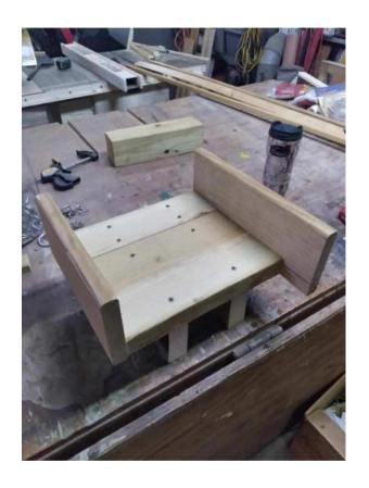
b) Using three 3½" deck screws, attach part 4 to the right side of the jug base, be sure all of the excess length is located beyond the front of the jug base.
